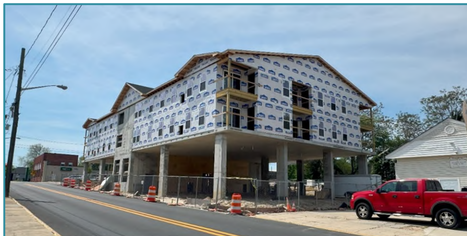
Figure 17: 118 North Central Avenue Construction
